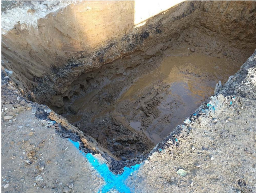
Photo 2. Septic Tank Excavation indicating running Sand and high groundwater level
