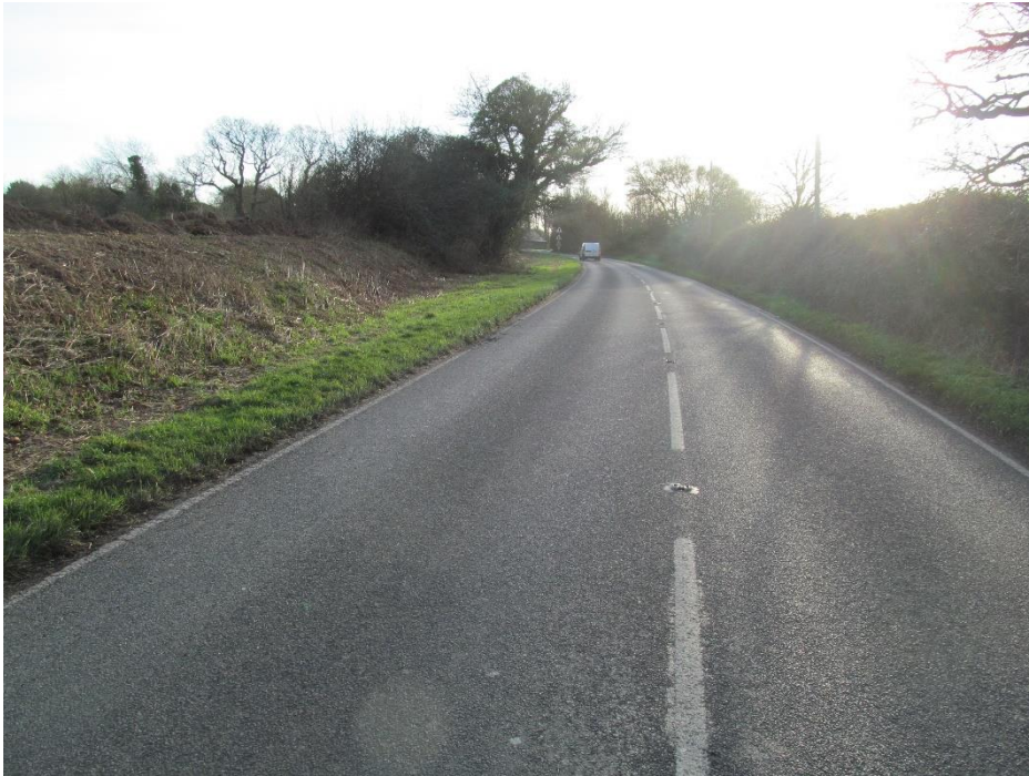
View from 120m looking south Bilsham Road.
