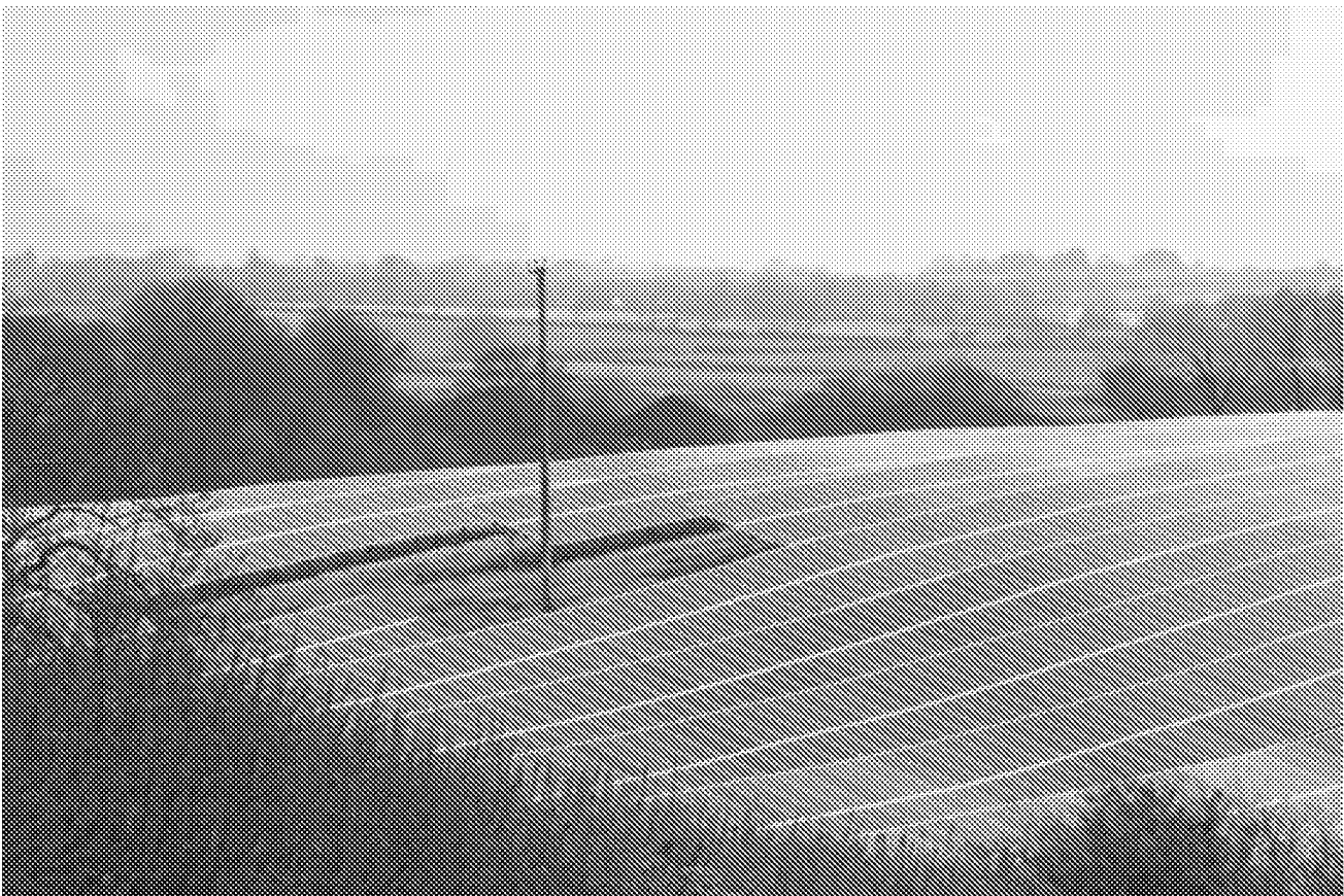
Figure 4: Example of solar panels following topography at Jordanstone Solar Park
