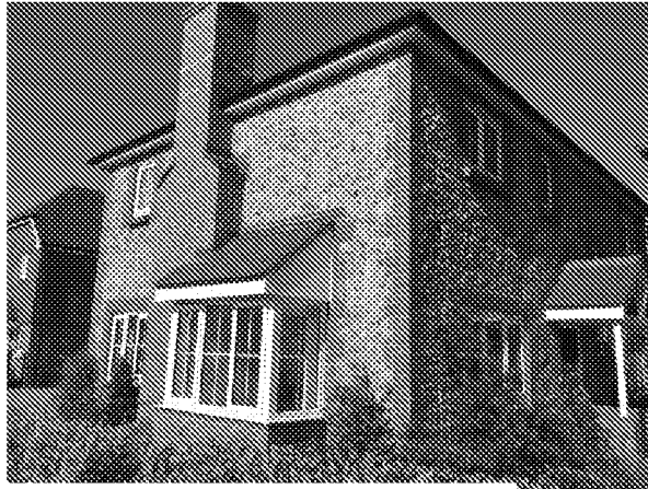
Example of flint block and decorative warnham red stock bricks
