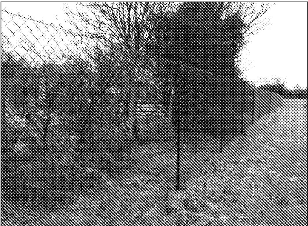
Chain-link on angle iron uprights
