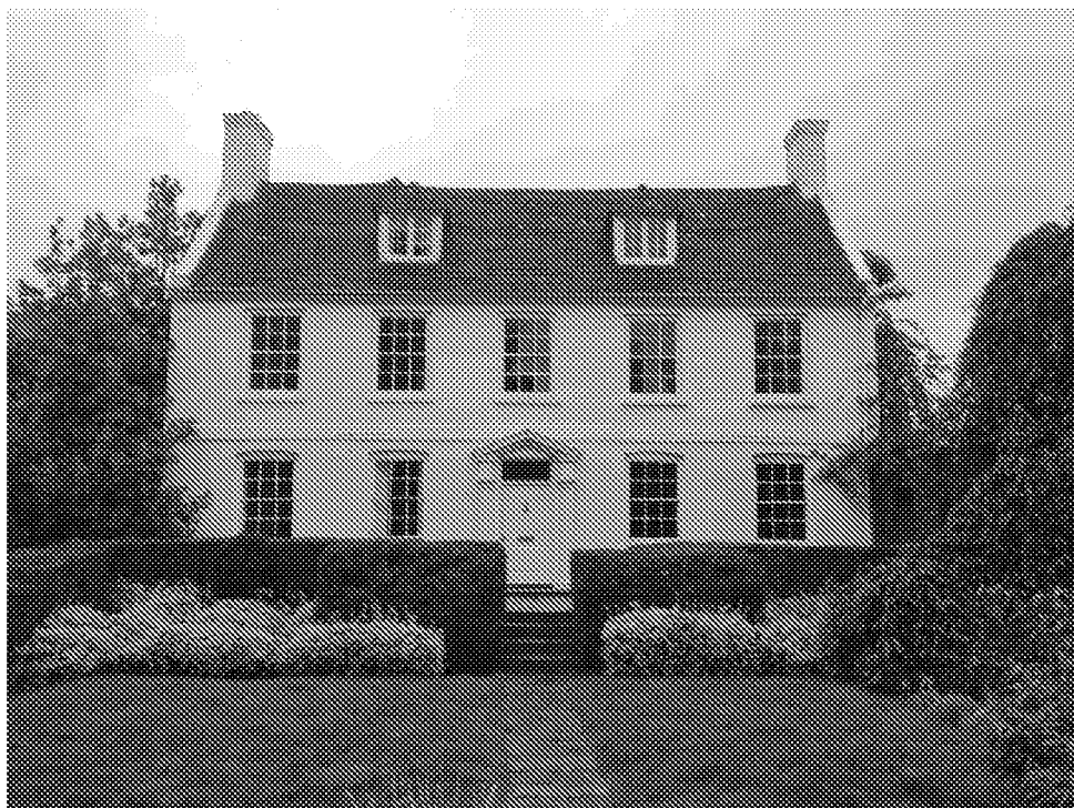
Fig No.1 – Image of Existing Front Elevation
