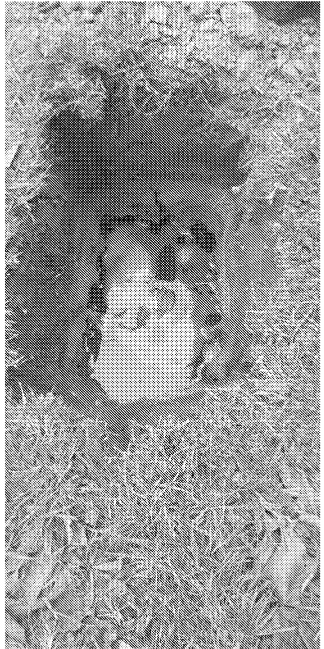
BRE 365 test pit
