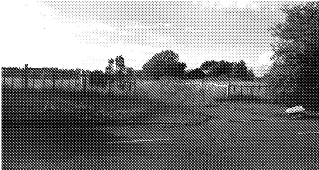
Figure 2.1: Existing Site Frontage and Access
