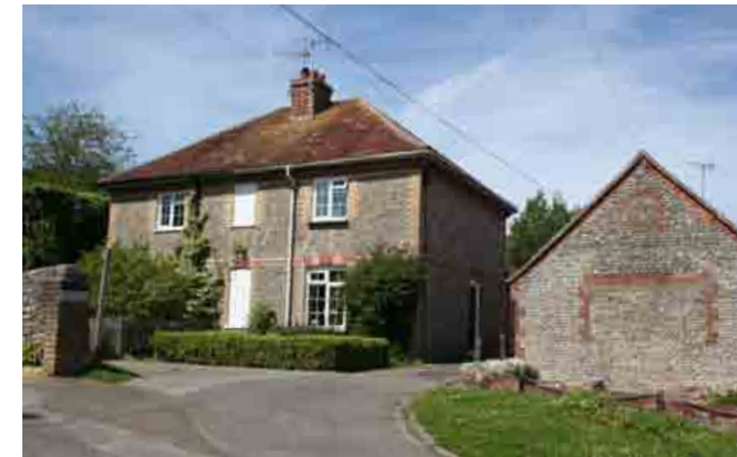
East and West Pound Cottages in the eastern part of the Conservation Area (Church Road)
