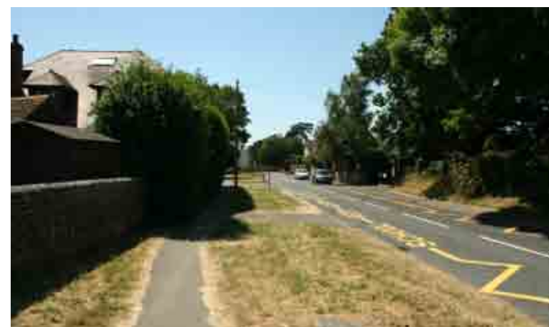
Footpath set behind wide grass verge
