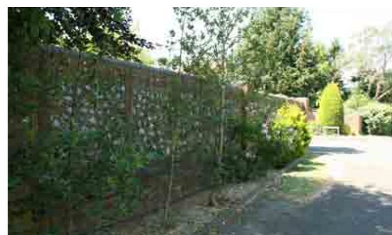
High brick and flint wall with planted verge
