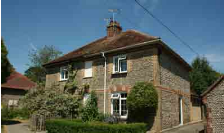
Flint elevations with brick string course and detailing
