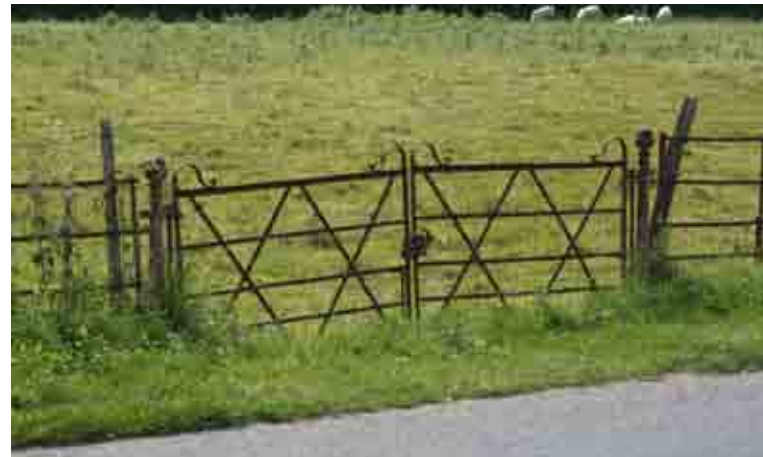
Iron fencing on Main Road to edge of site
