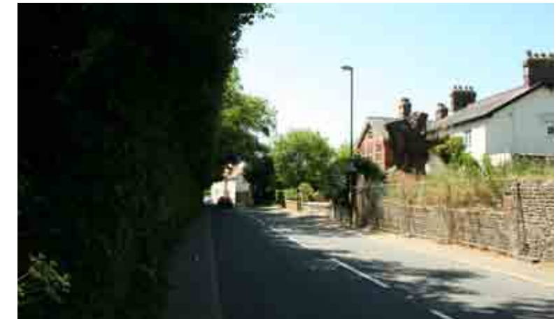
North End Road with high boundaries against the back of footway
