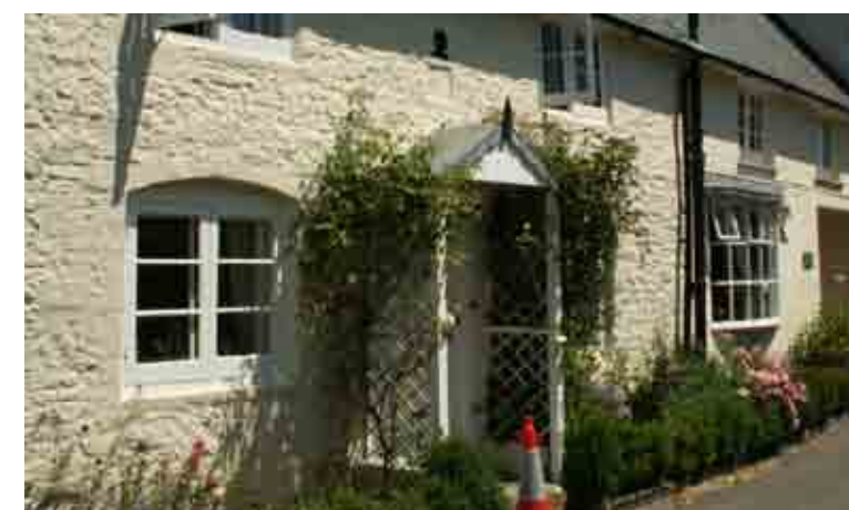
Open porch with trellis in Church Road
