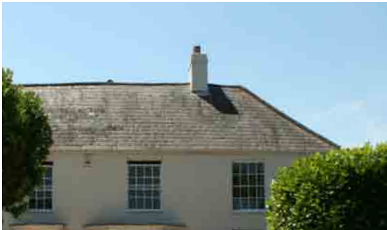
Fully hipped roof in Church Lane
