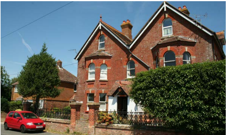
Red brick in Church Road
