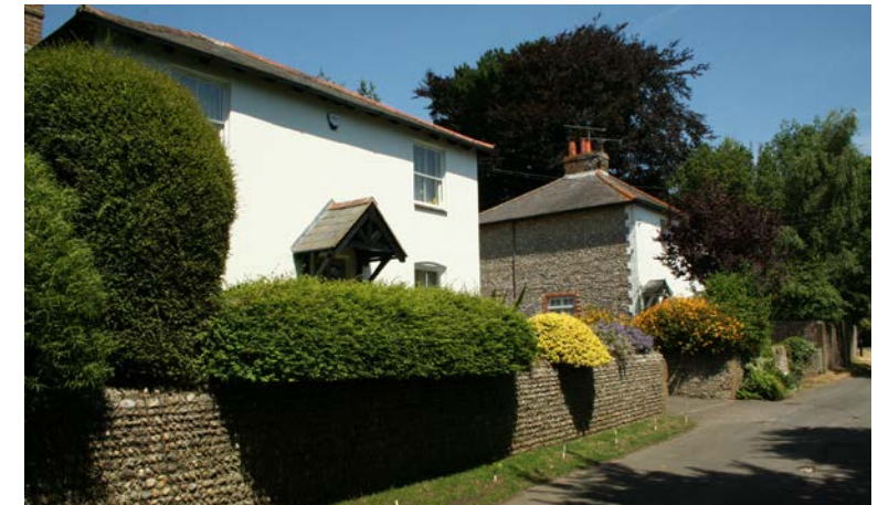
White painted cottage in Church Lane set back behind a wall
