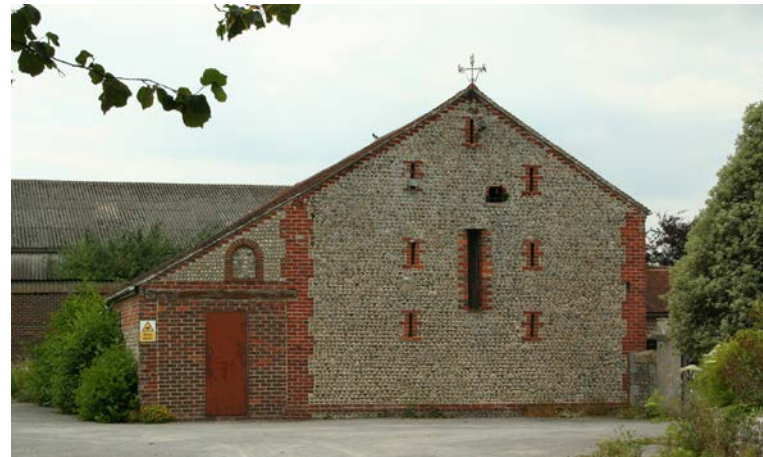
Brick and flint barn at Stakers Farm
