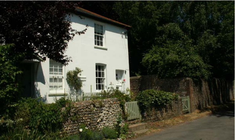
Pair of Two Bay Semi detached houses in Church Road
