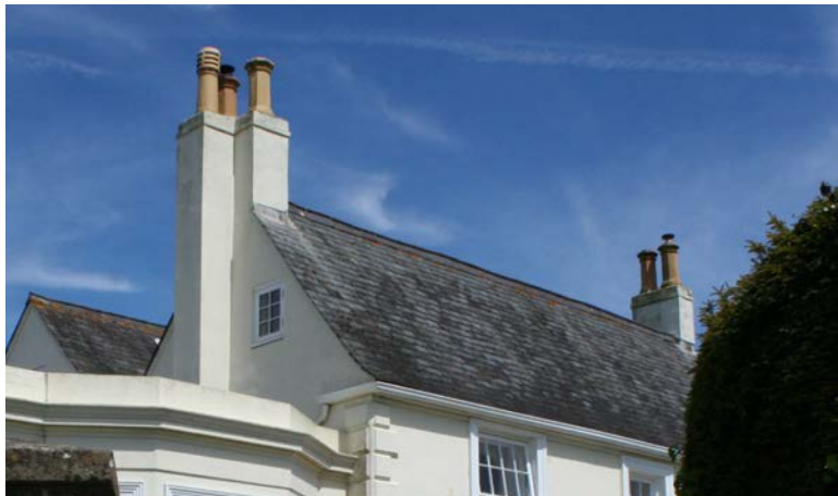
Gabled ended roof at Bonhams Farmhouse with no barge boards
