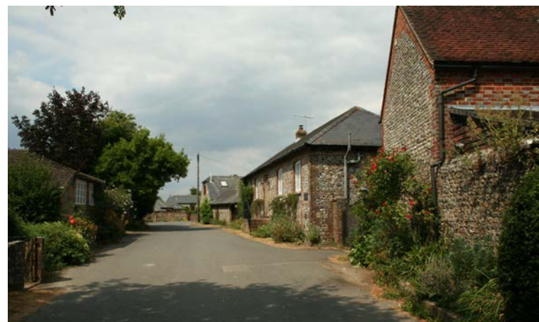
Hoe Lane in Flansham with converted agricultural buildings
