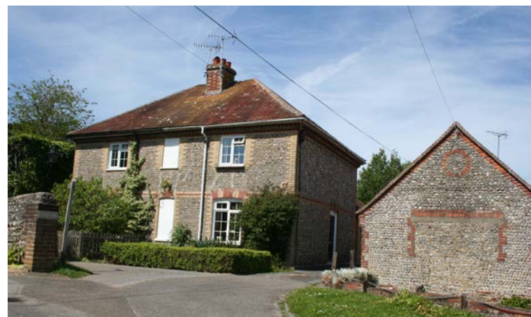
Flint housing in Church Road with brick detailing
