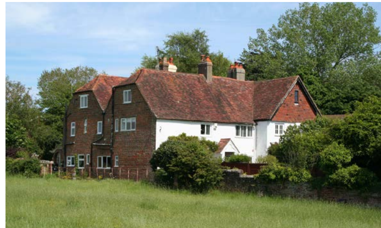
Laburnum Cottages in the Conservation Area with brick and render
