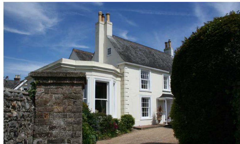
Bonhams Farmhouse (white stucco)
