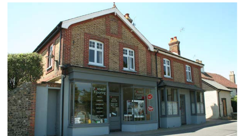
Contrasting brick elevations in Main Road
