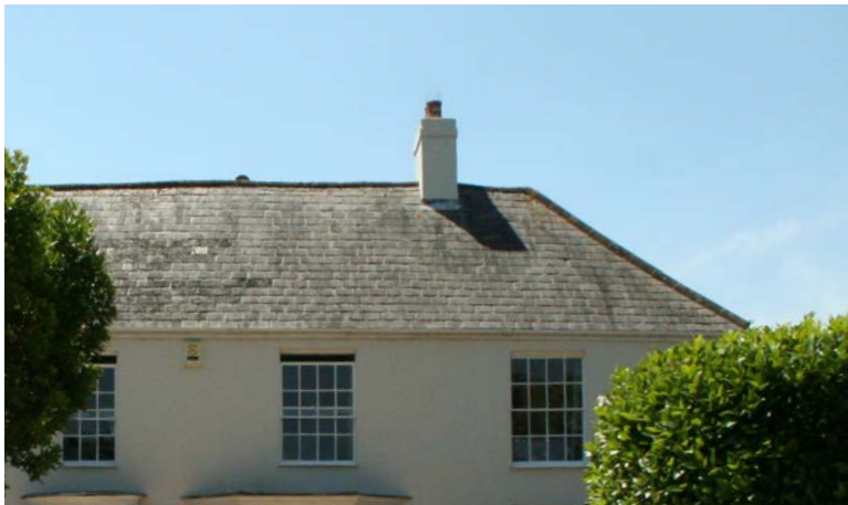
Fully hipped roof in Church Lane
