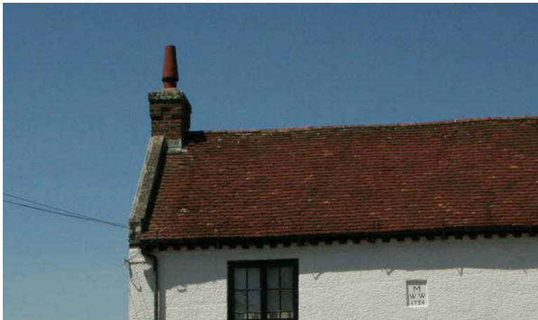
Plain clay roof with brick corbel detail and parapet gable end
