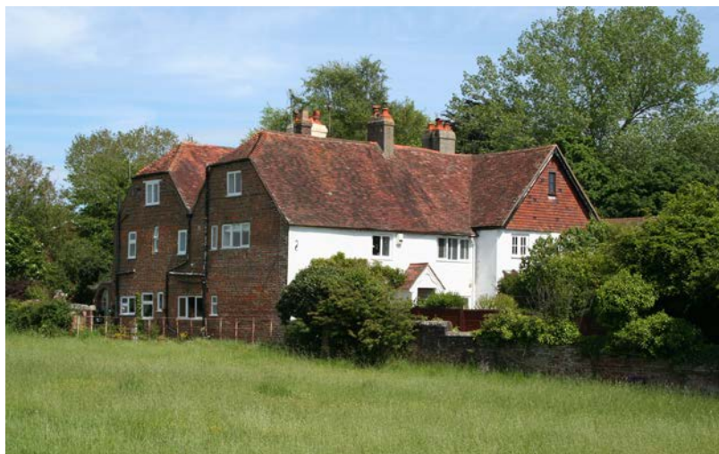
View across the Conservation Area from Main Road looking east towards Laburnum Cottages (Grade II)
