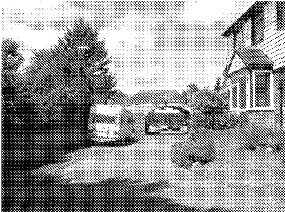
Figure 28: The Old Canal Bridge, running over the old Portsmouth to Arundel Canal
