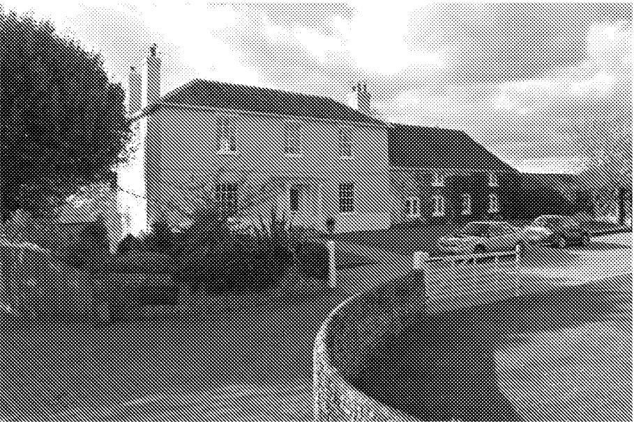
Figure 40 Bilsham Manor showing two distinct phases of development
