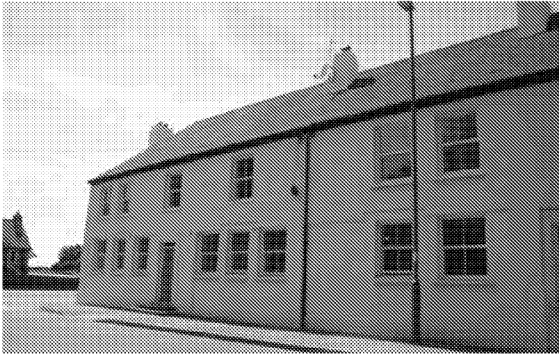
Recently refurbished cottages on the junction of Main Road and North End Road
