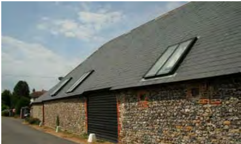
Flint elevations with red brick detailing and dark painted timber boards on converted barn in Flansham
