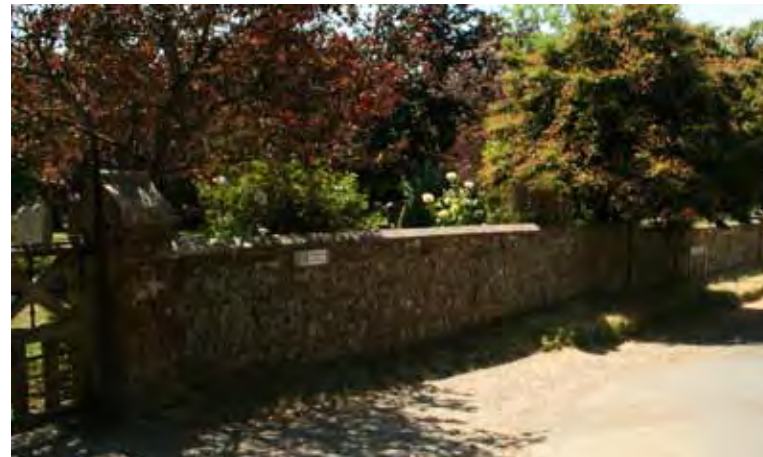
Low walls and narrow verges in Church Road
