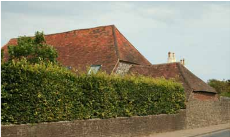
Half hipped plain clay tiled roof at Bonhams Barn
