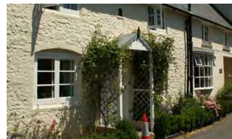
Open porch with trellis in Church Road
