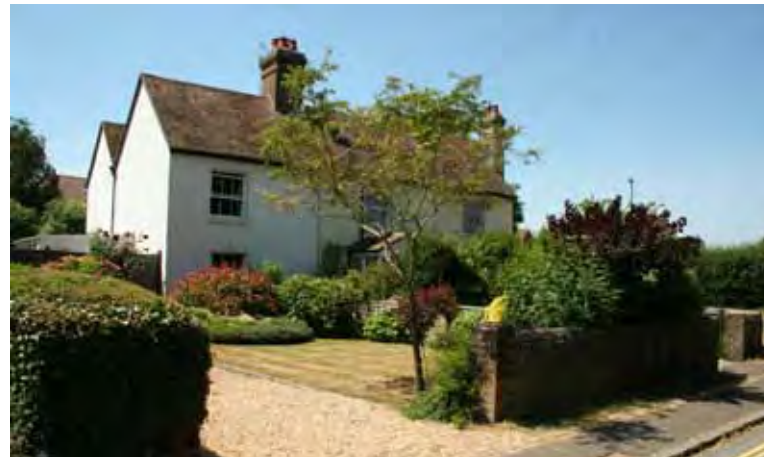
Church Lane with footway, narrow verge and brick wall
