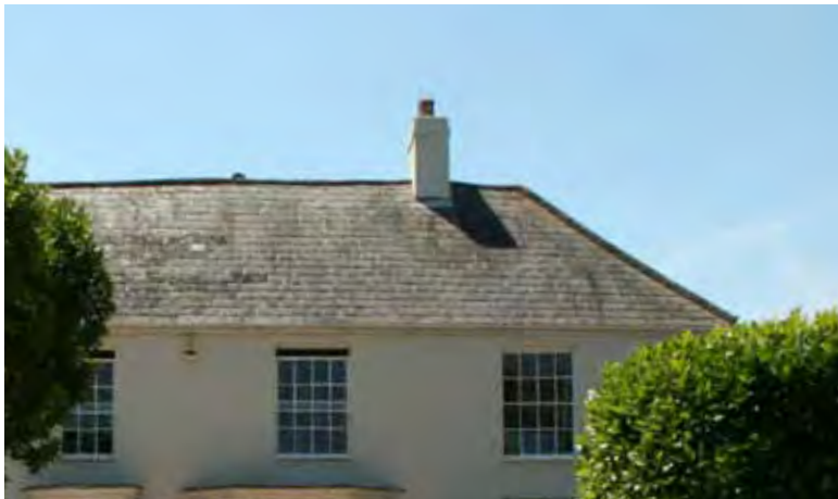
Fully hipped roof in Church Lane
