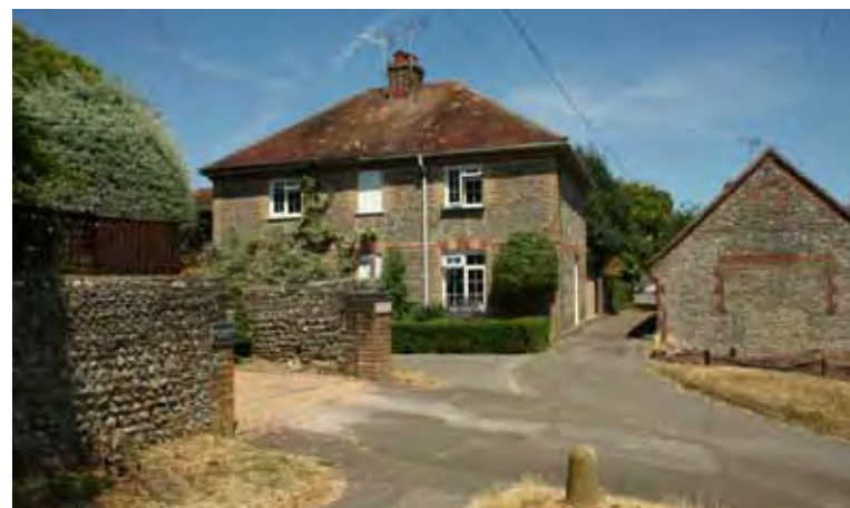
Church Road with shared surfaces
