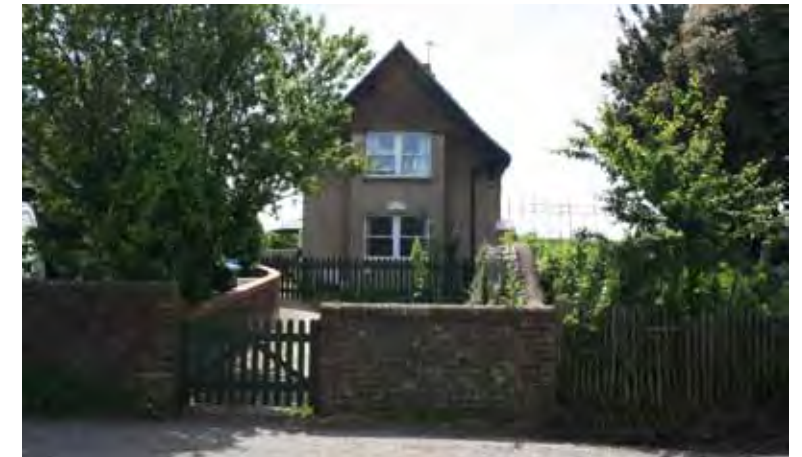
Timber gate with brick / flint wall in Conservation Area next to site
