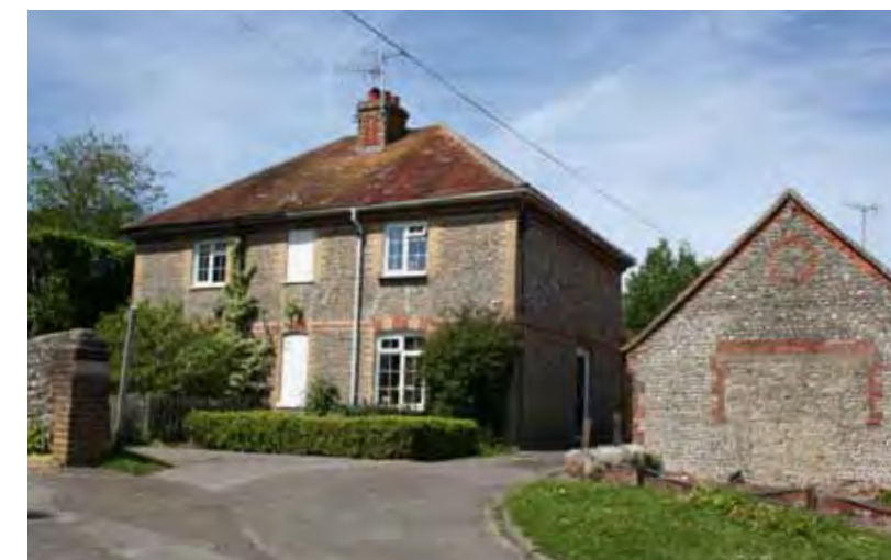
East and West Pound Cottages in the eastern part of the Conservation Area (Church Road)
