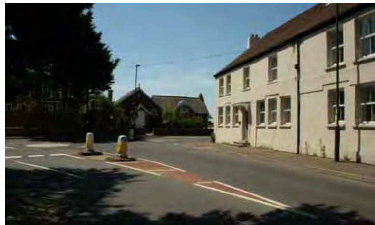
Building in North End Road directly at back of footway
