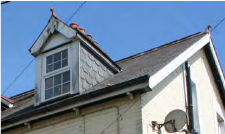
Pitched dormer in roof of property in Bilsham Road
