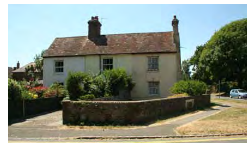
Boundary walls with footway set behind grass verges in Church Lane
