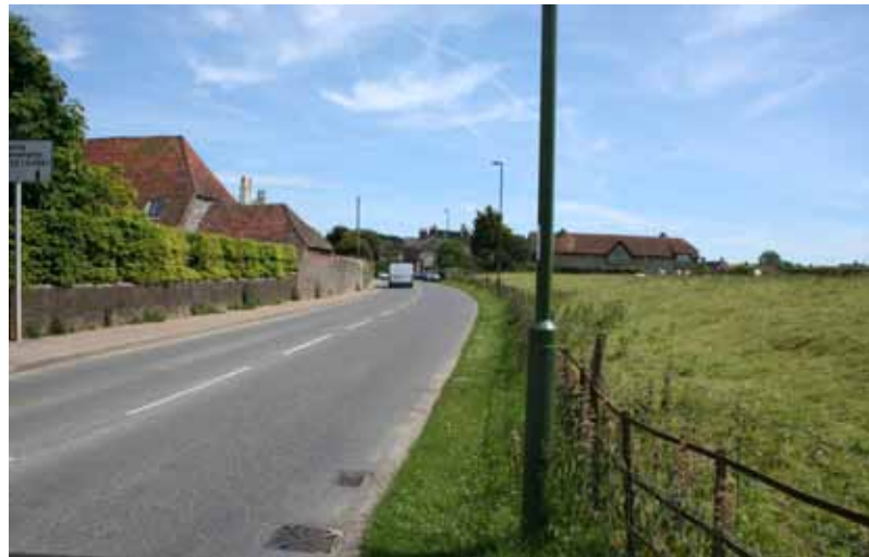
View looking east along Main Road with the open field and Conservation Area left and Bonham's Barn (Grade II) right.
