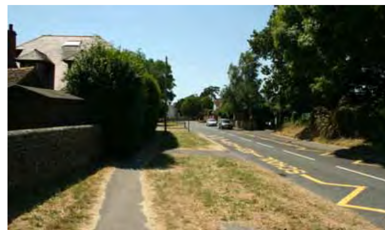
Footpath set behind wide grass verge
