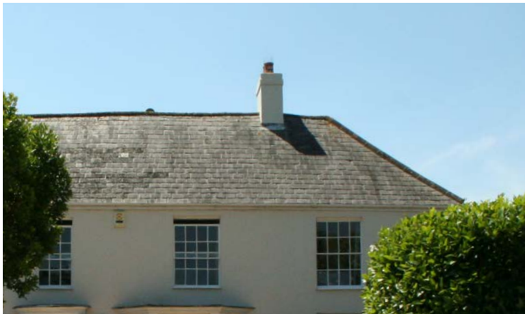
Fully hipped roof in Church Lane
