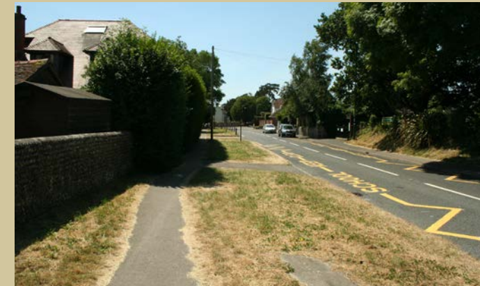
Footpath set behind wide grass verge
