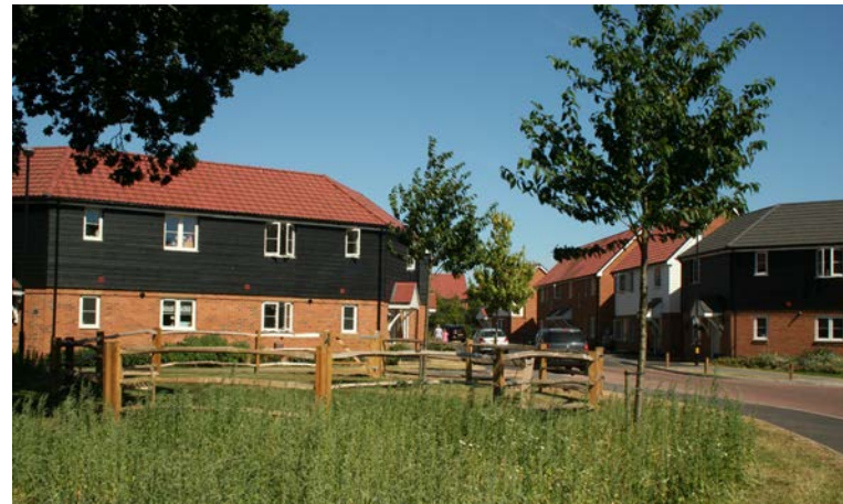
Recent housing in Navigation Drive
