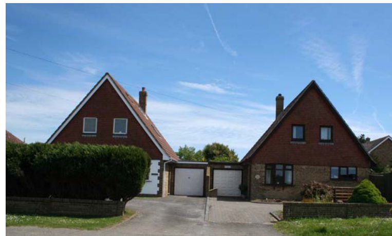
Pair of linked buildings in Bilsham Road
