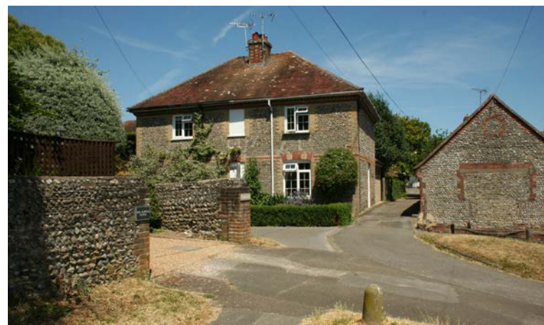
Church Road with shared surfaces
