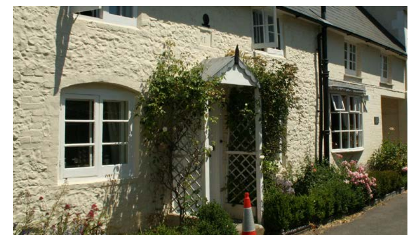
Open porch with trellis in Church Road
