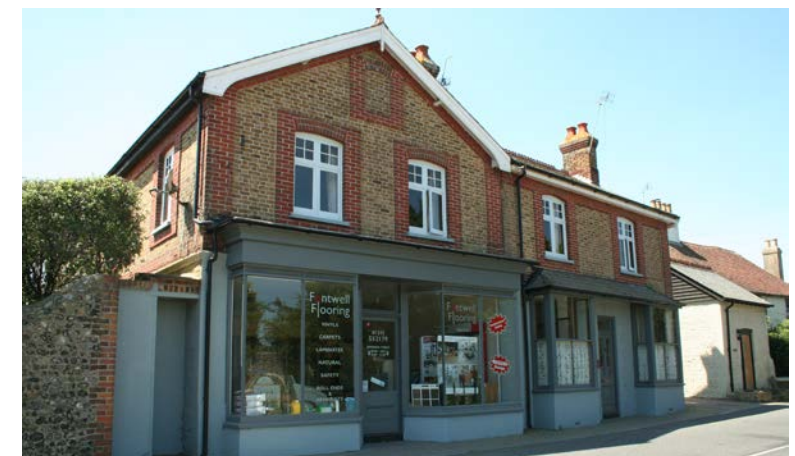
Contrasting brick elevations in Main Road
