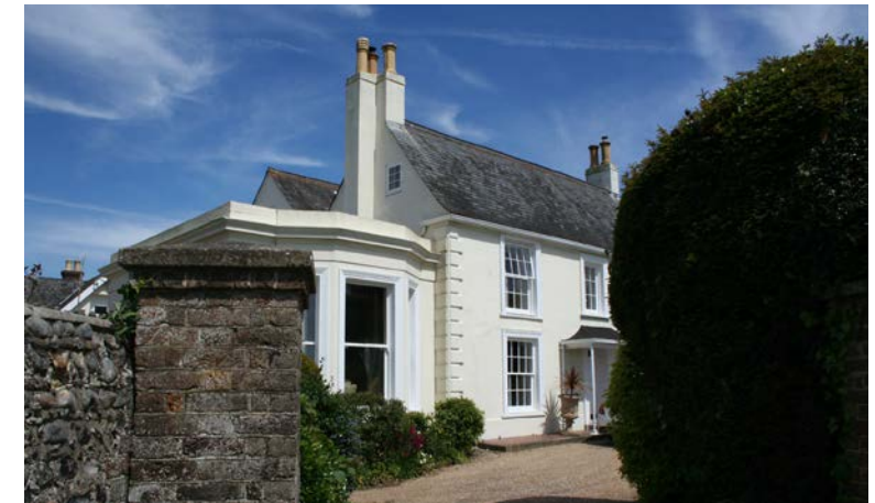
Bonhams Farmhouse (white stucco)
