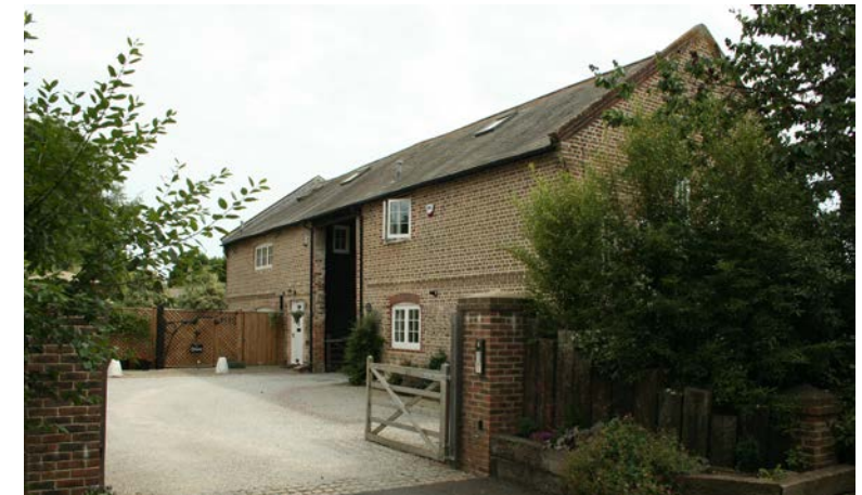
Converted barns at Hobbs Court
