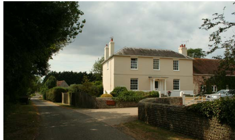
Bilsham Manor with a range of brick and flint outbuildings
