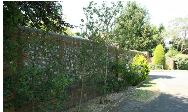
Tall brick wall with flint inset panels in Church Lane
