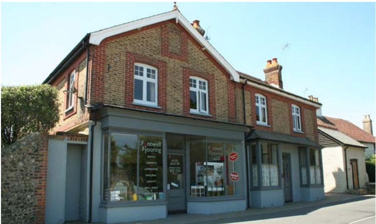
Yellow brick with and red brick ornamentation in Main Road
