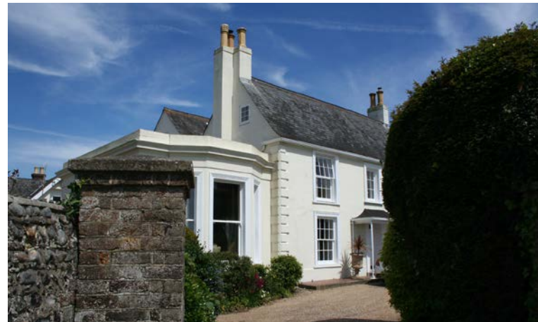
Bonhams Farmhouse (white stucco)
