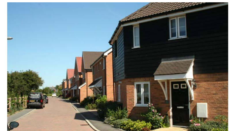
Housing in The Towpath with a consistent building line
