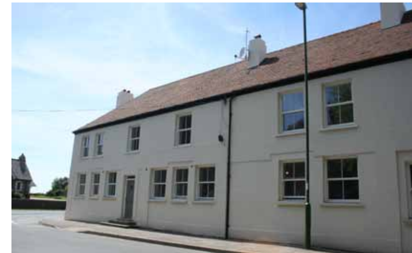
Recently refurbished cottages on the junction of Main Road and North End Road
