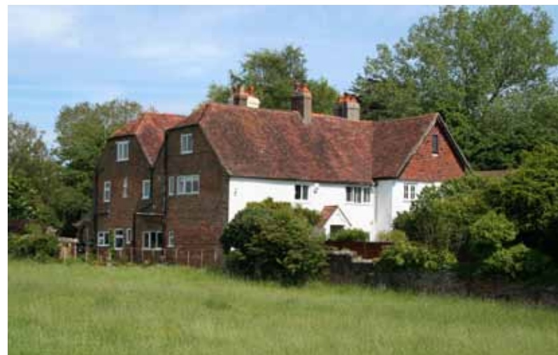
View across the Conservation Area from Main Road looking east towards Laburnham Cottages (Grade II)
