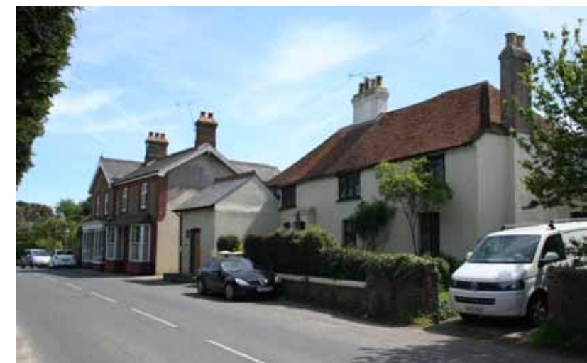
View east along Main Road with properties in the Conservation Area with short gardens or directly addressing the street
