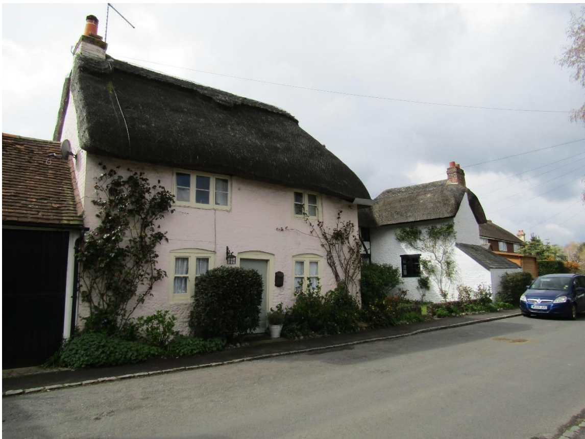
Figure 7 -full elevation of listed building
