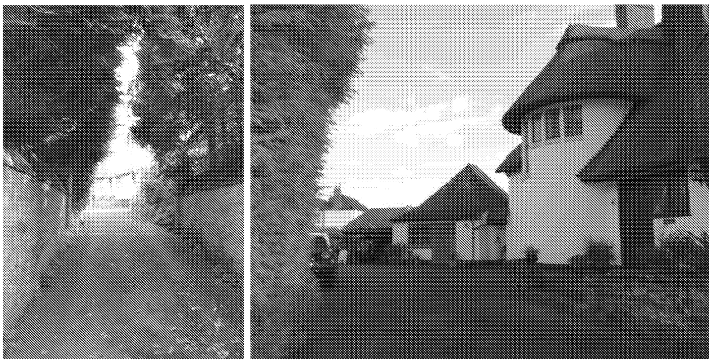
(Photos 3/4 - Driveway and approach to house from the main road)
