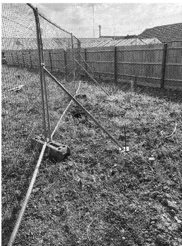
Photograph 6 – Updated and current tree protection rear of plot 6
