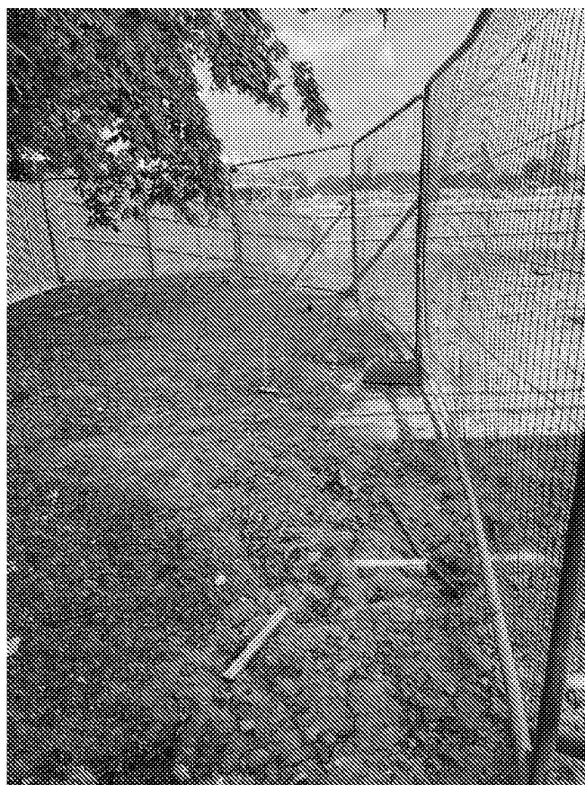
Photograph 4 – Updated and current tree protection rear of plots 1 and 2
