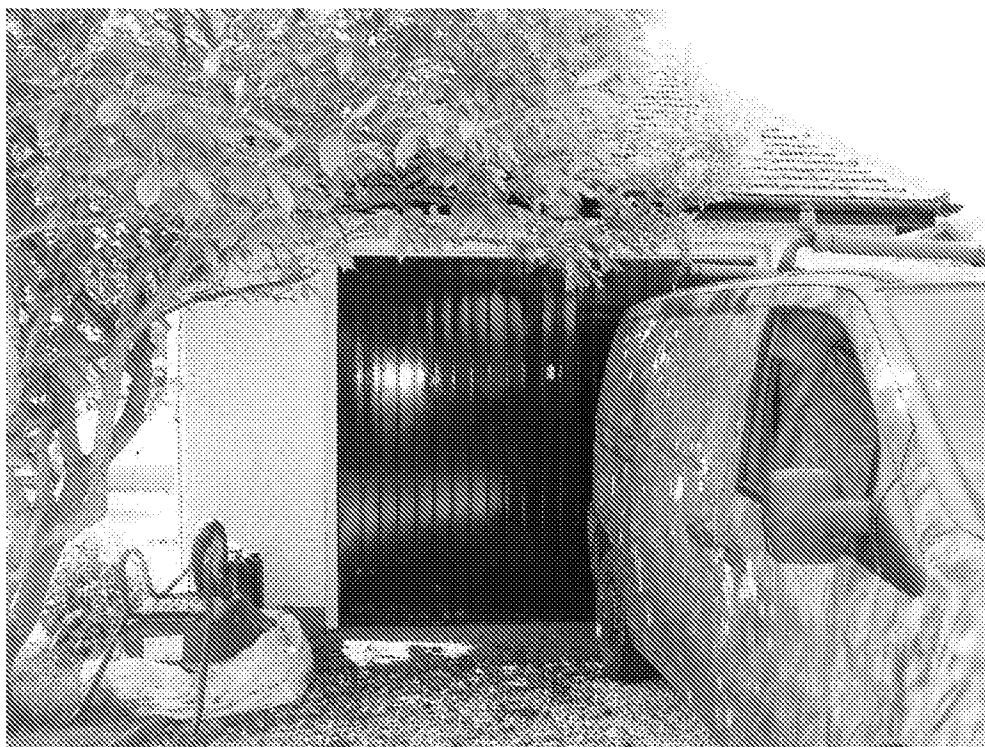
Photograph 2. Front elevation of the garage (Northern elevation).
