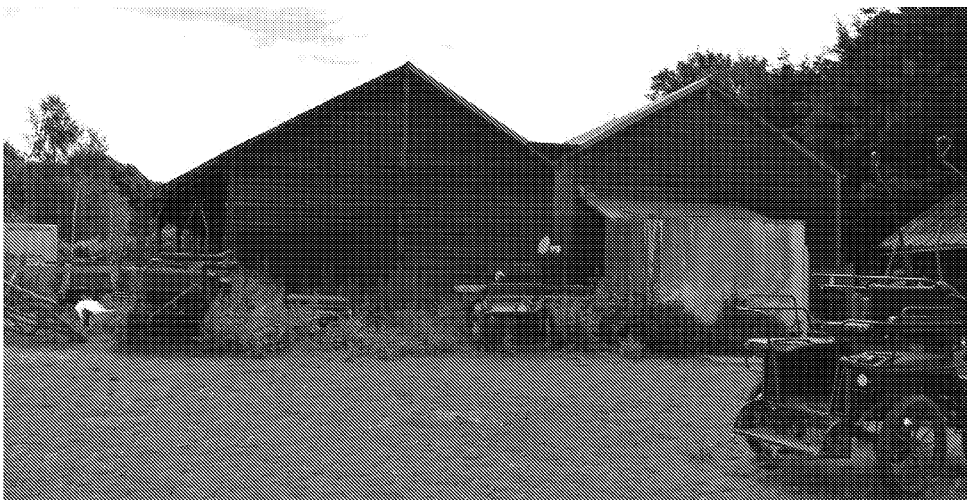
Photograph No. 04 - Building 1, western aspect of the double barn.
