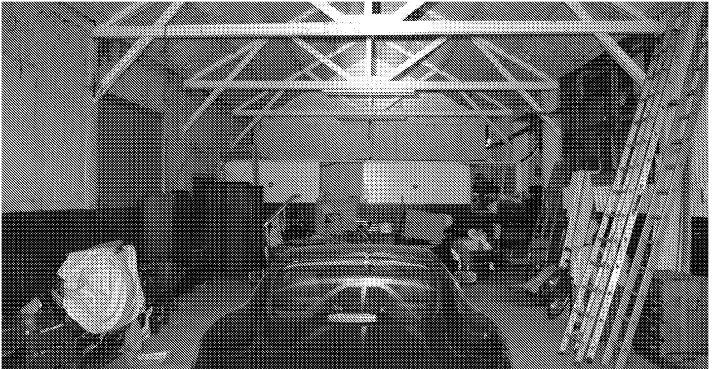
Photograph No. 05 - Building 1, internal view of section 1. Exposed rafters, tightly sealed to wooden panels.
