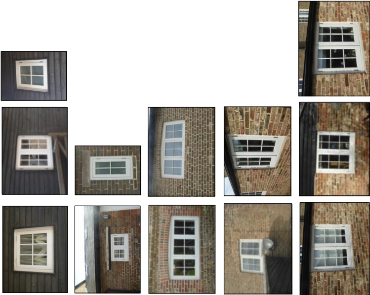
IMAGES OF EXISTING EXTERNAL WINDOWS
