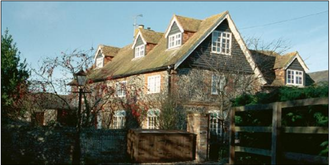
Two-and-a-half-storey Traditional Dwelling within Flansham
