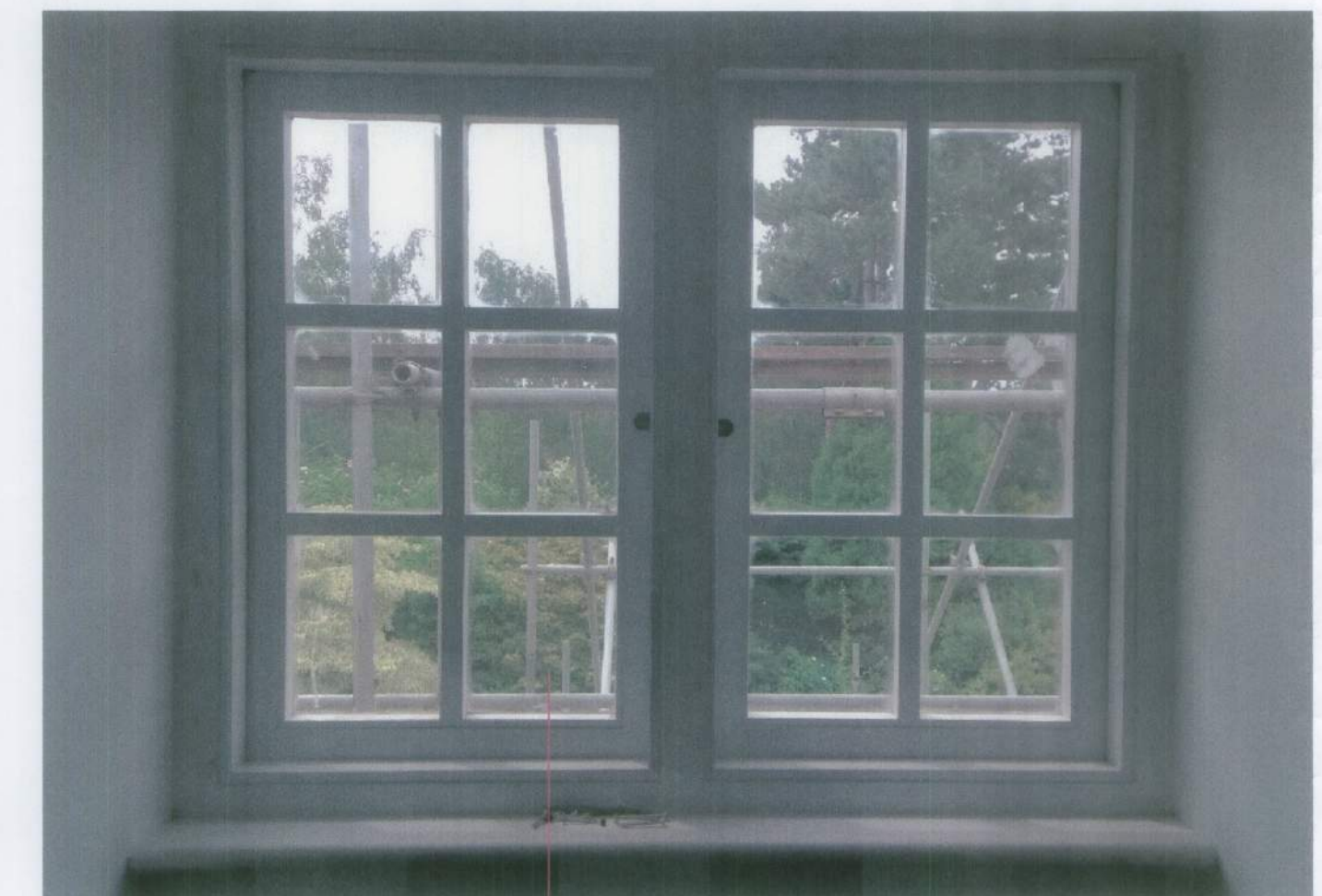
Replaced Window as Built
