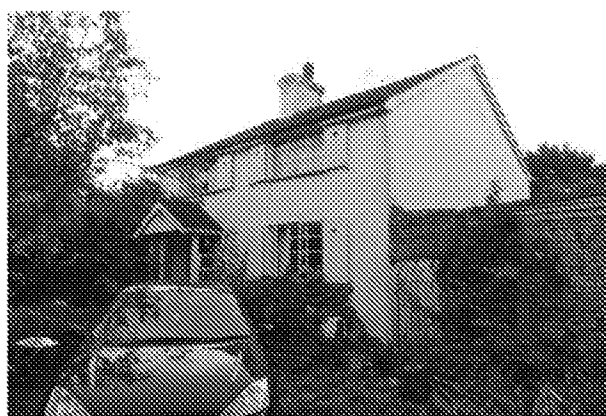
Image 2: The existing North (front) elevation of 'old house'
