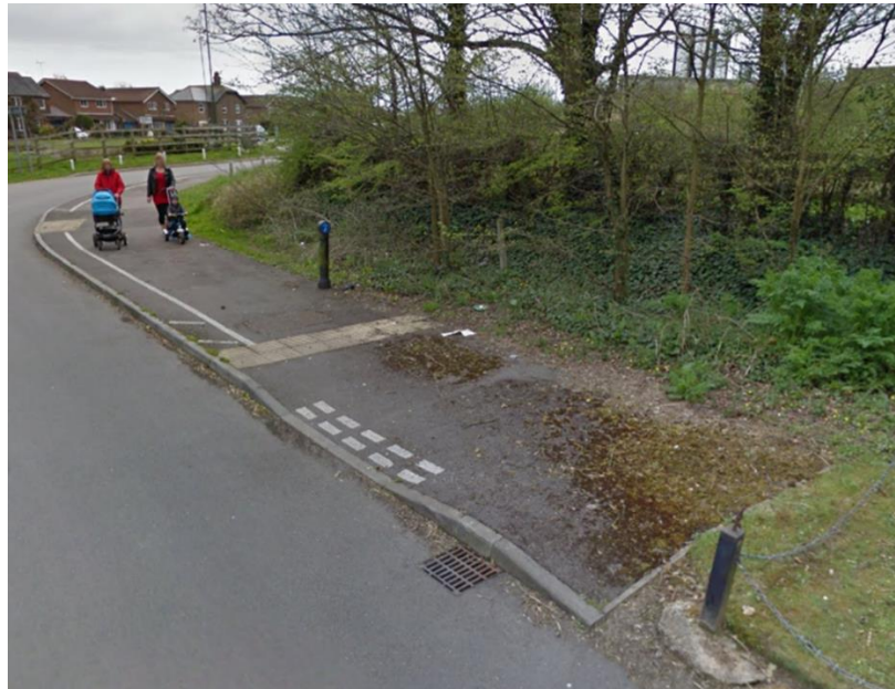
Figure 2.6: Pedestrian Footway Flanking Hoe Lane
