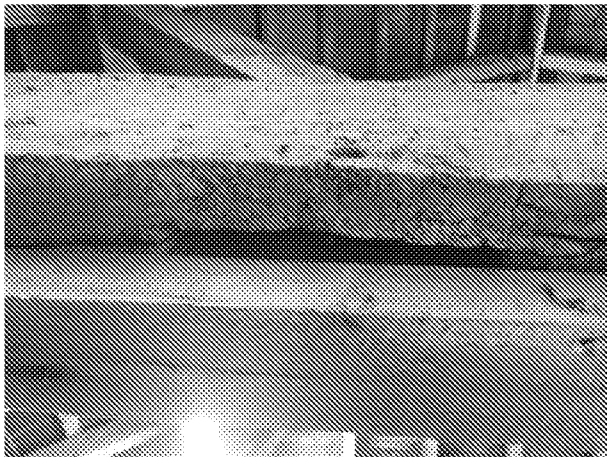
Old mortice tenon joint partly obstructed by modern timber.
