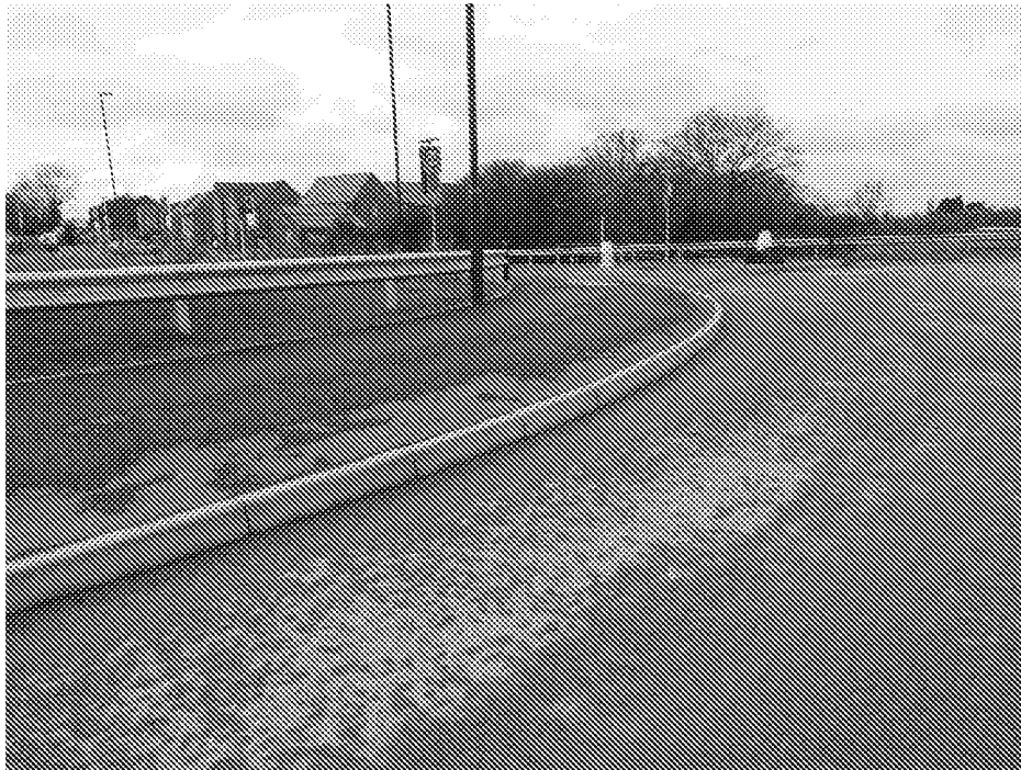
NRR westbound lane approaching the Southern Arm of the Stanover Lane Roundabout.
