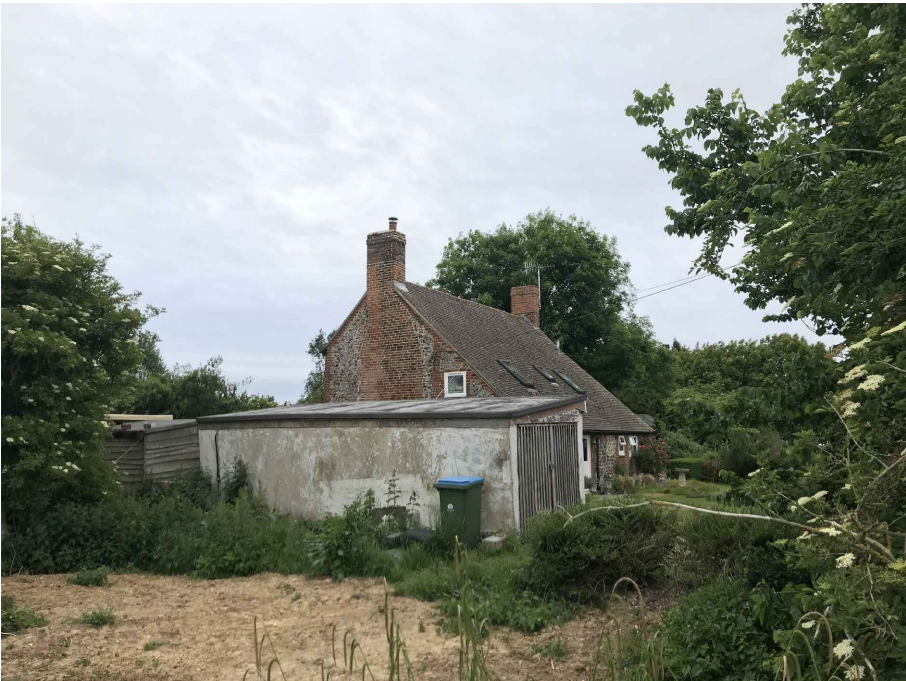
LOOKING SOUTH EAST
