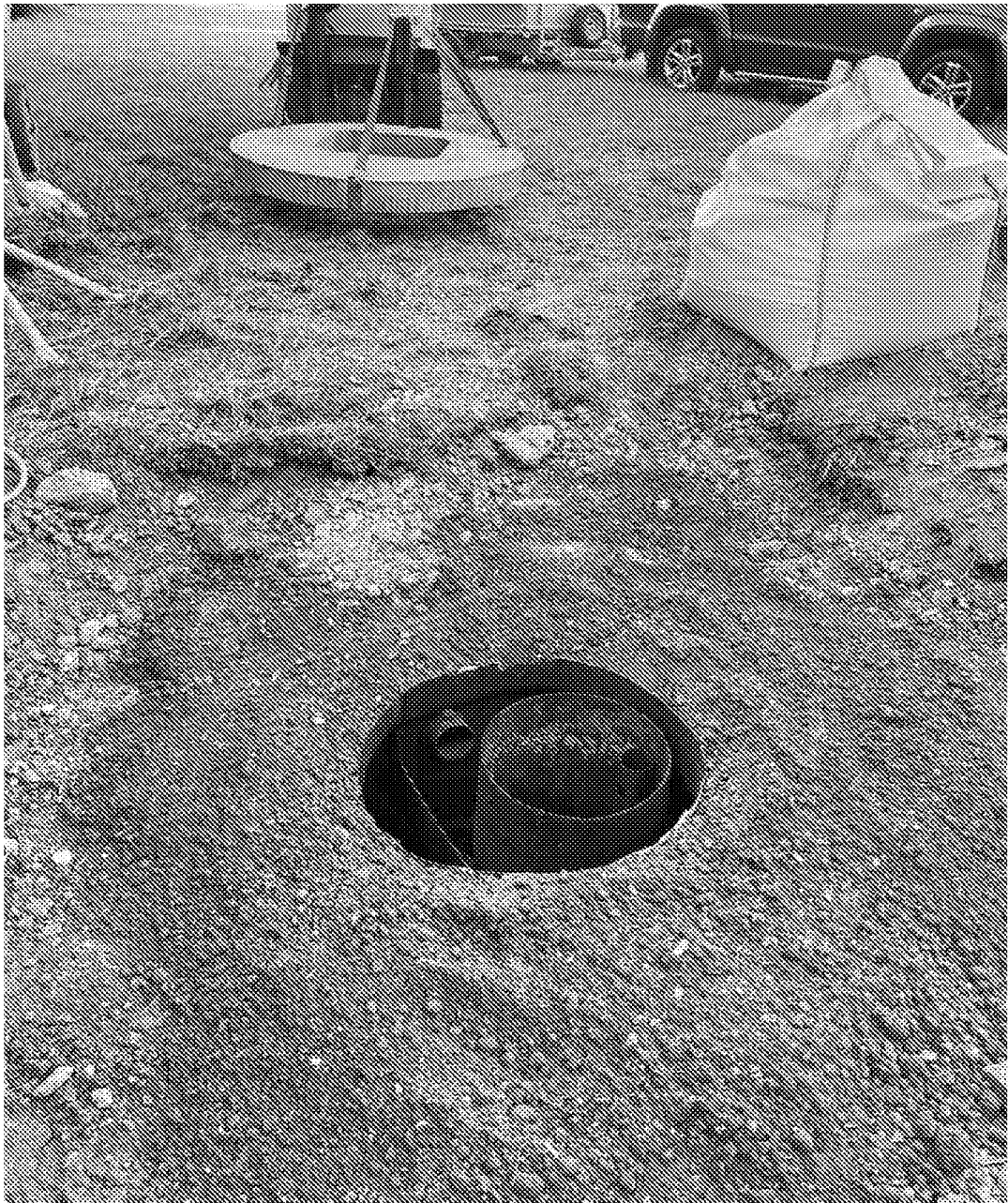
Photograph 15: OWI repair works (August 2020)
