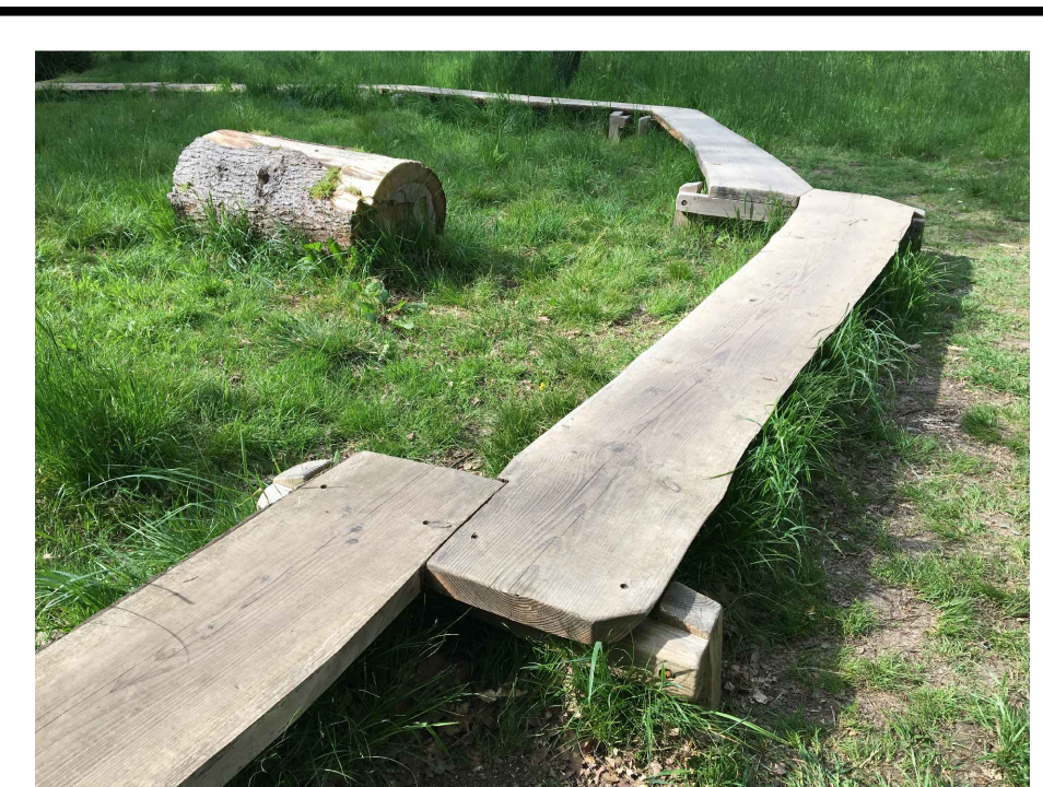
Hardwood balancing beams to create a path over meadow
