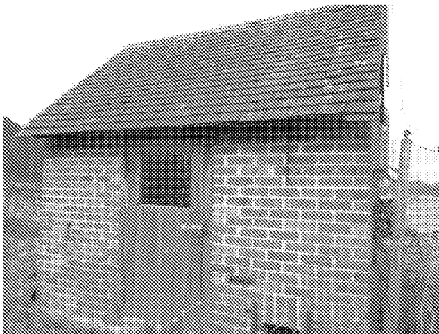
Building B3: External view, south-east aspect.
