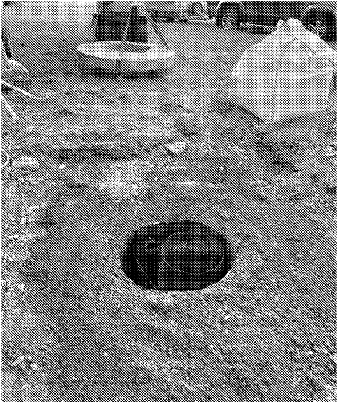
Photograph 15: OWI repair works (August 2020)
