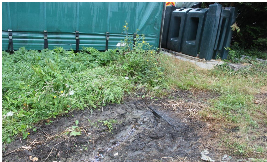
Photograph 14 Leaking OWI just south west of the employment area, waste oil tank in the background
