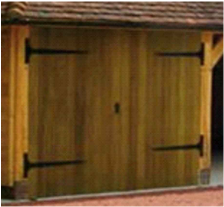
COVERED PARKING DOOR STAINED BLACK
