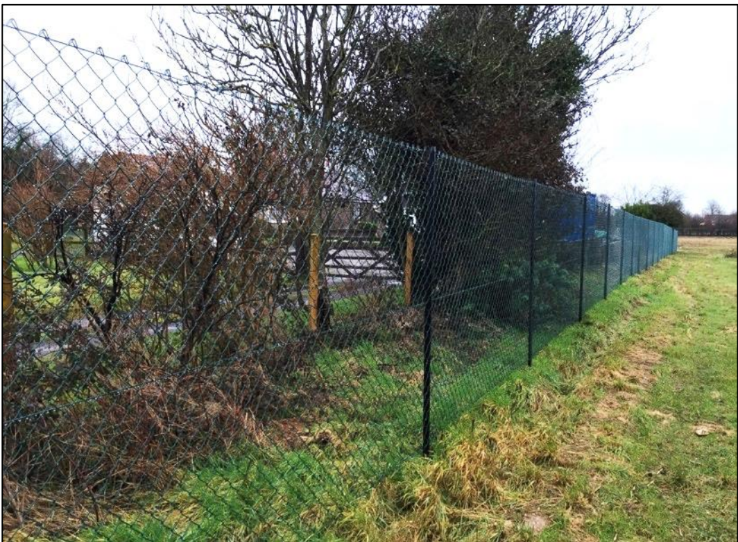
Chain-link on angle iron uprights
