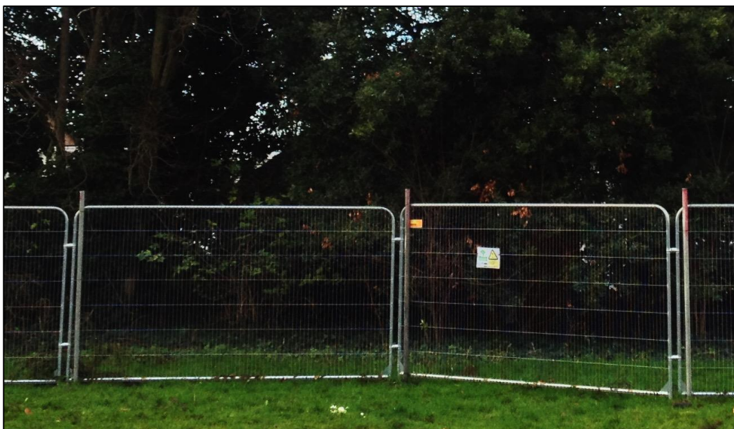
Weld-mesh panels on scaffold uprights
