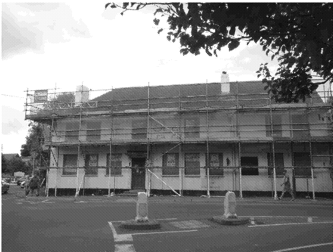
Plate 15: The Olive Branch Public House
