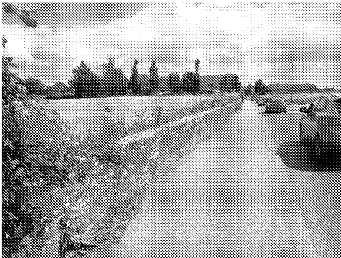
Plate 1: Coped wall marking site's south western boundary with road into Yapton
