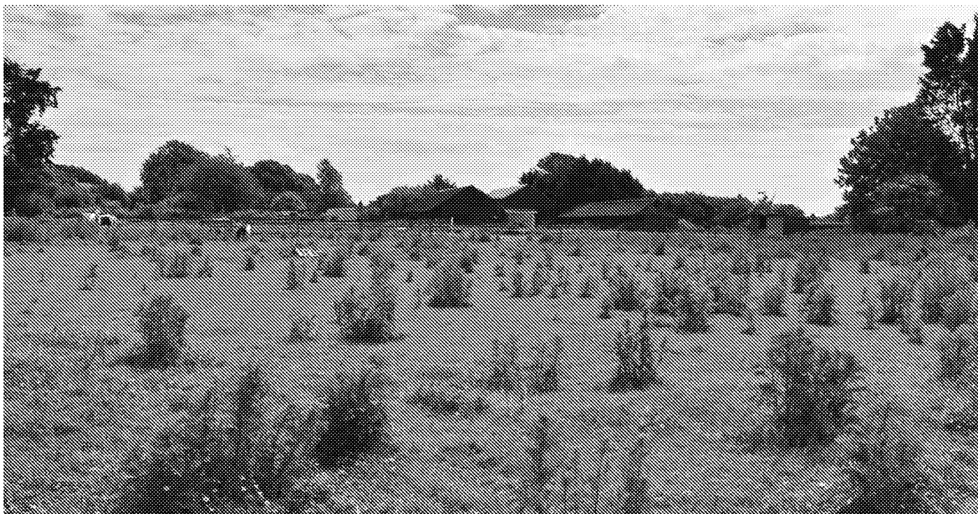
Photograph No. 01 - Northern aspect of all buildings on site and surrounding paddock.
