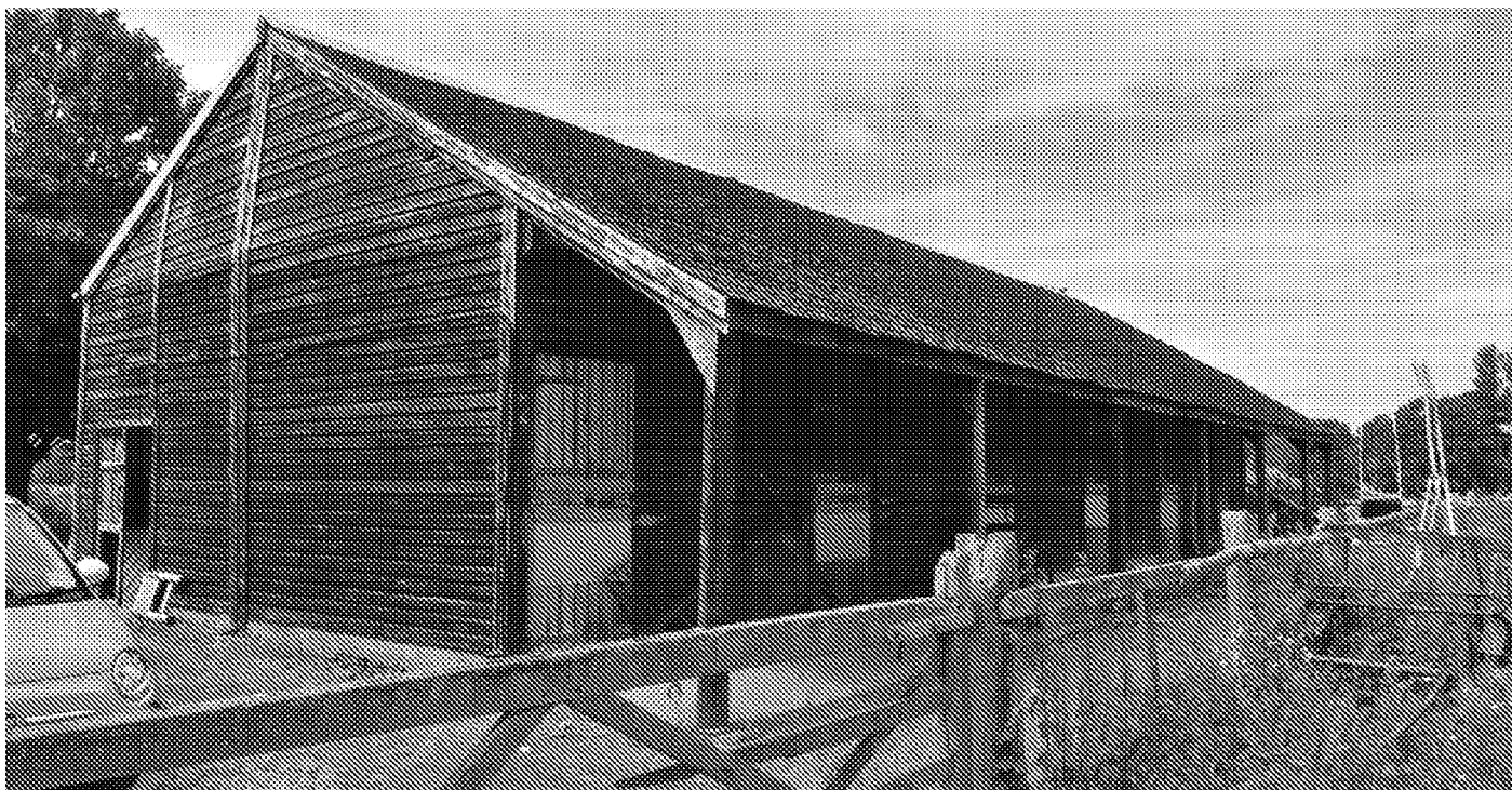
Photograph No. 03 - Building 1, Northern aspect, stable door access points not in use.
