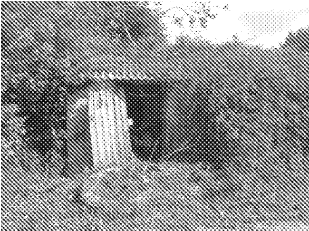
Photo 9. Building 5 southern aspect, following clearance of dense scrub.
