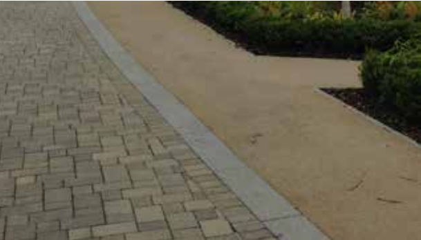
Tactile shared surface
