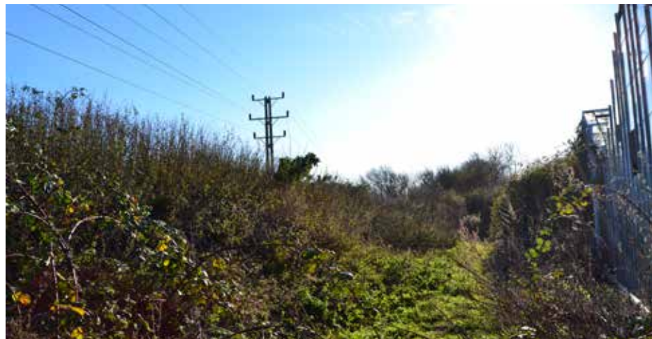
4. Electricity lines and western boundary
