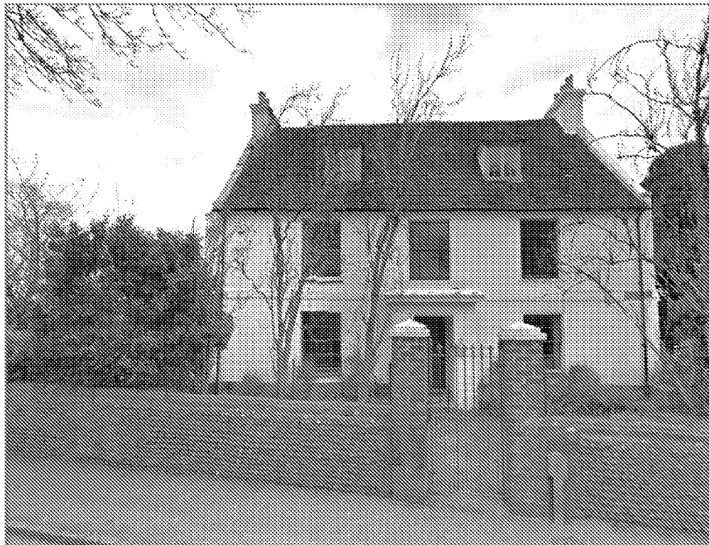
Figure 1 – Front of Stakers Farmhouse
