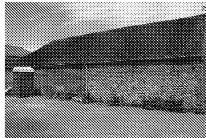
Figure 6 – Barn 1 south elevation
