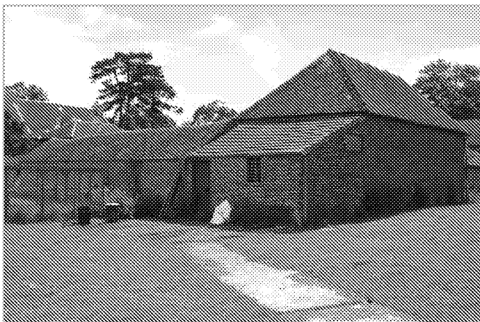
Figure 9 – North elevation to Barn 2 and stable building
