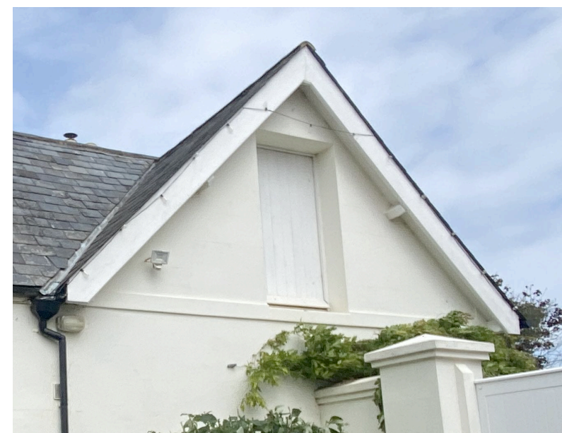
Stable door - first floor gable
