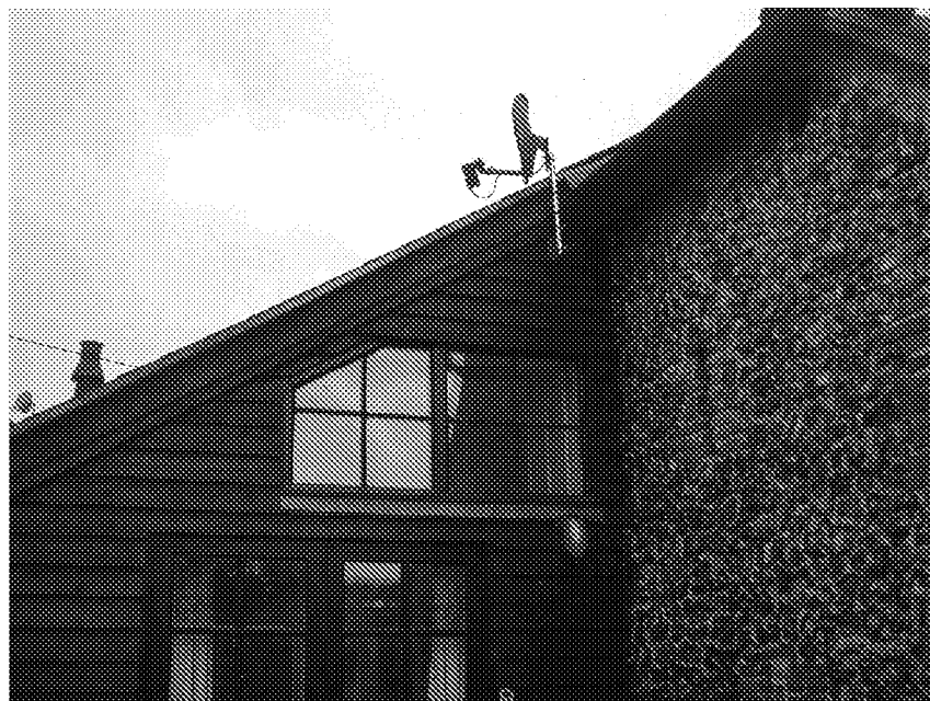
Picture – Part of the rear elevation of Wellow Barn with stained cedar weatherboarding.
