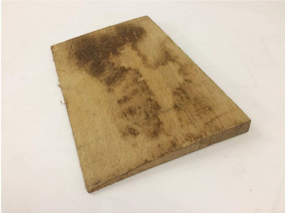
1.7 – Oak weather board [also representative of the oak fascia board]
