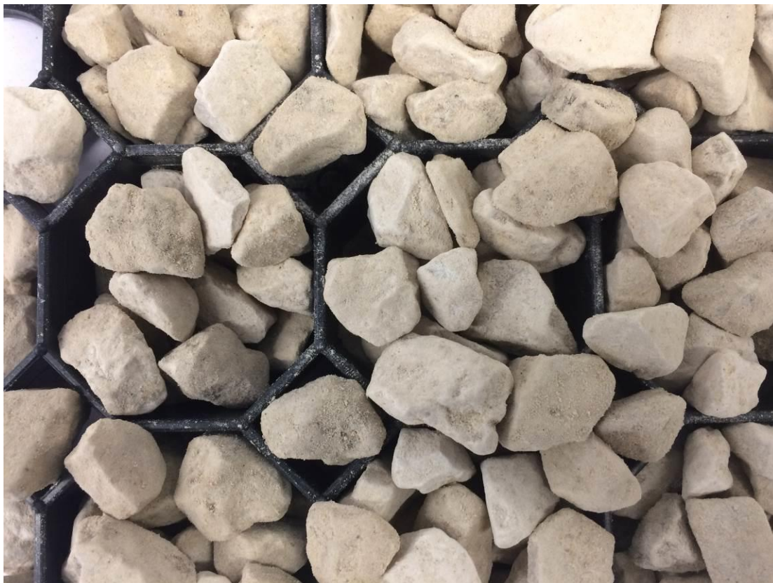
1.11 – BodPave gravel retention system with 'cotswold stone' [view from above]
