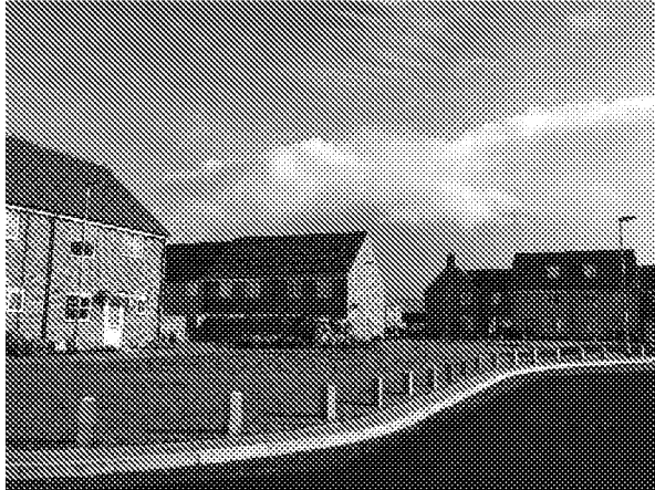
Figures 3 and 4. Images of a swale along the road on a site in Fordham (Img. Swale01 and Swale02) demonstrating how a carefully designed swale can form a key part of a Public Open Space scheme
