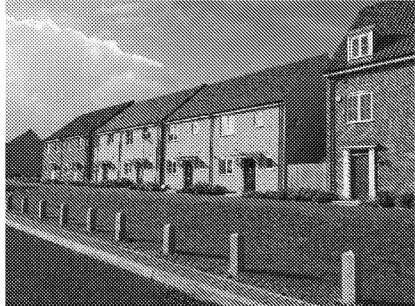
Figures 3 and 4. Images of a swale along the road on a site in Fordham (Img. Swale01 and Swale02) demonstrating how a carefully designed swale can form a key part of a Public Open Space scheme
