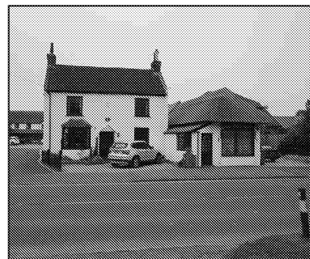
Photograph R - Listed building The Homestead, including attached outbuildings
