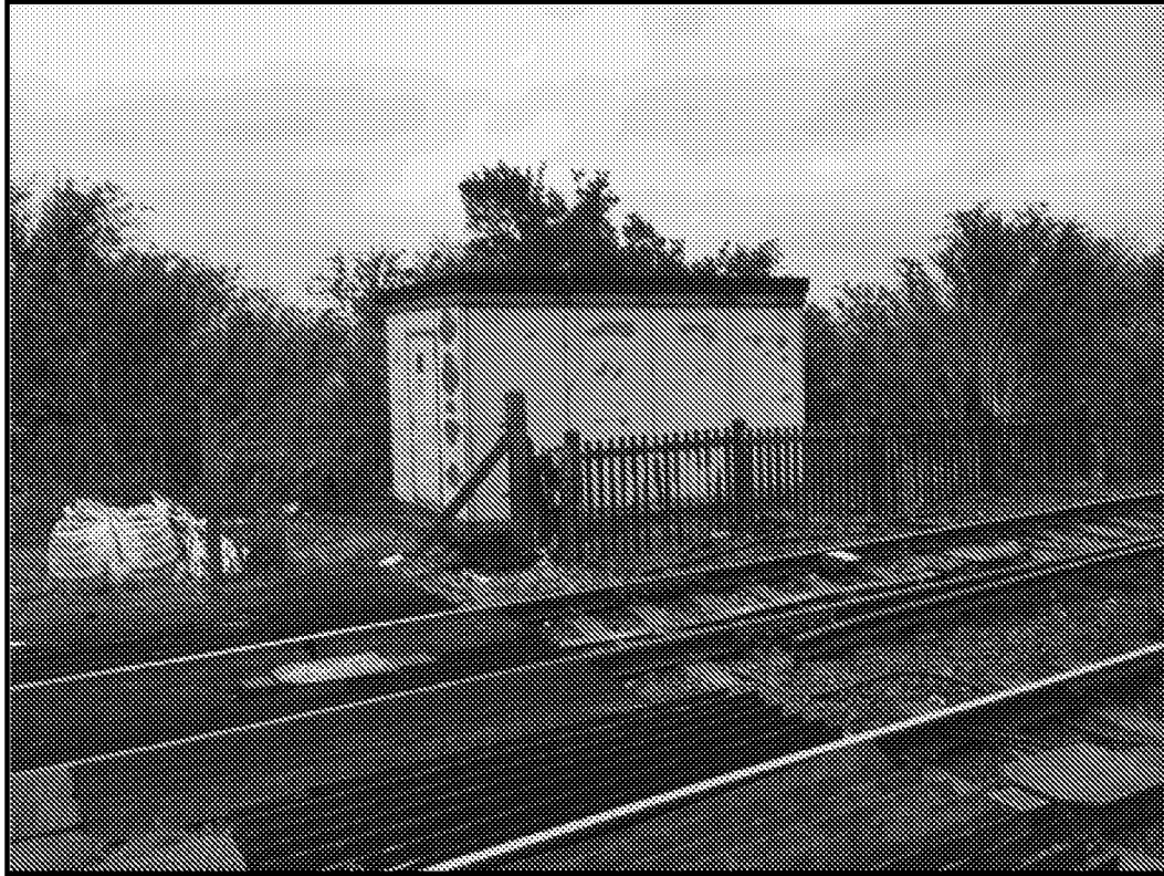
Figure 2: Existing REB Yapton Level Crossing
