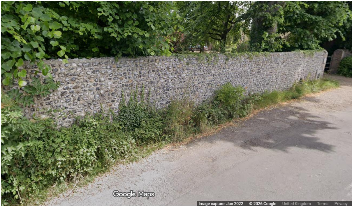
Extract from Google Street view circa June 2022 – Showing the impacted wall insitu.
