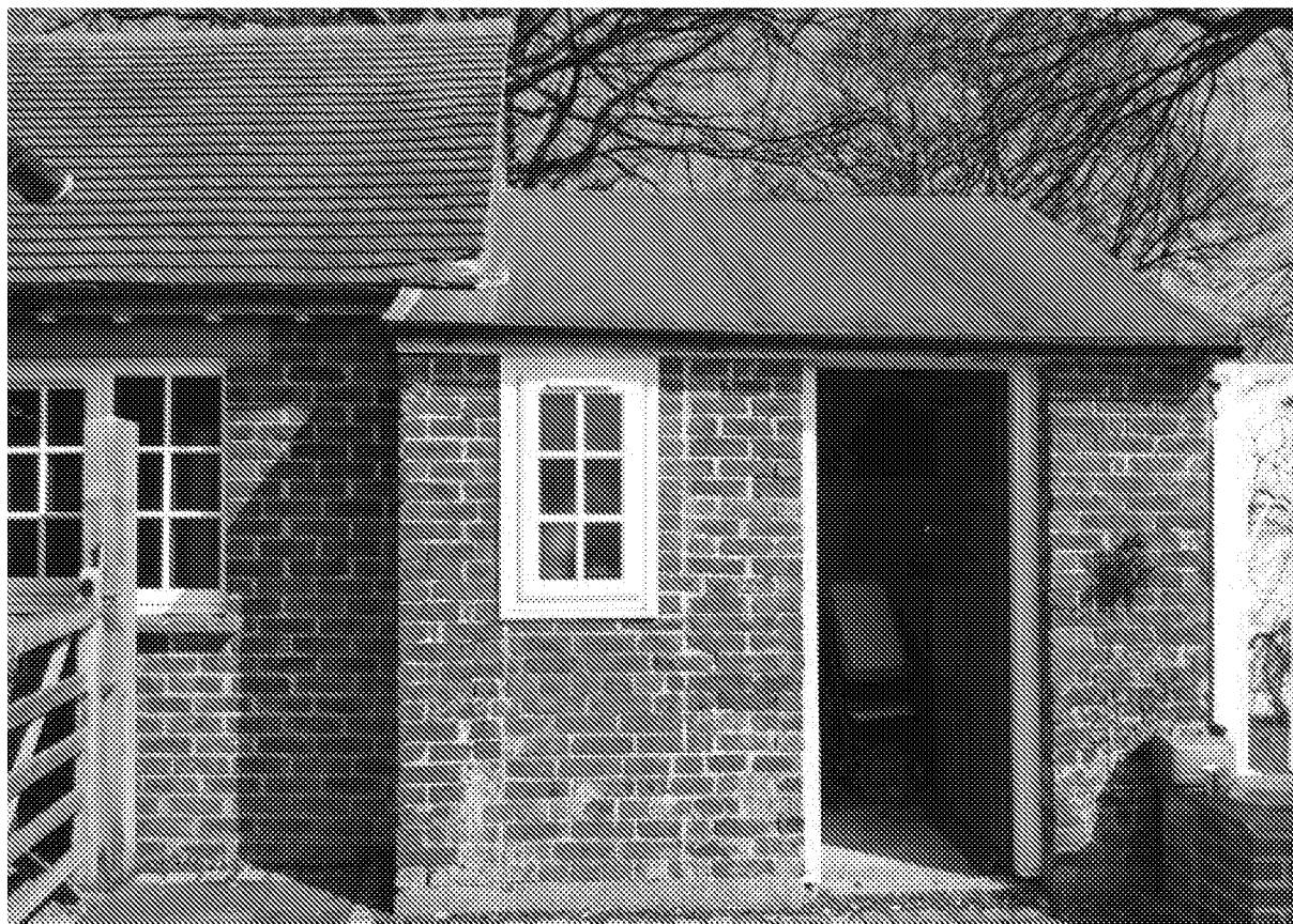
Figure 17. Brick built garage/outhouse with a tight fitting factory formed tiles are a section lined with bitumen.
