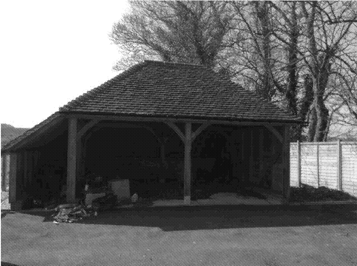
Figure 13. The newly built barn style shed located south of the southern property.
