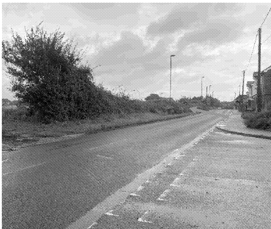
The proposed priority junction north of Taylors Close, taken from Taylors Close looking north-eastwards along the B2132 Bilsham Road.
