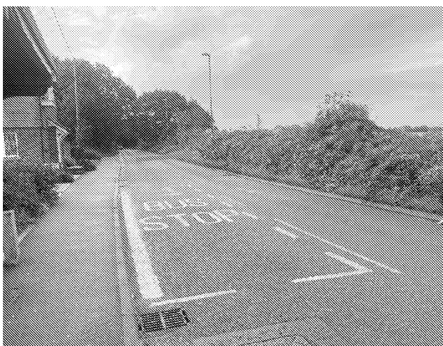
The proposed priority junction north of Taylors Close, taken from the B2132 Bilsham Road, looking south-westward. The location of the proposed vehicular access is arrowed.
