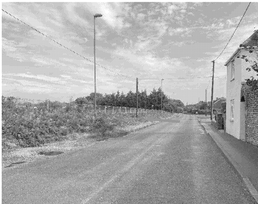
The proposed priority junction south of Graham Road, taken from the B2132 Bilsham Road, looking north-eastwards. The site of the new access is arrowed.
