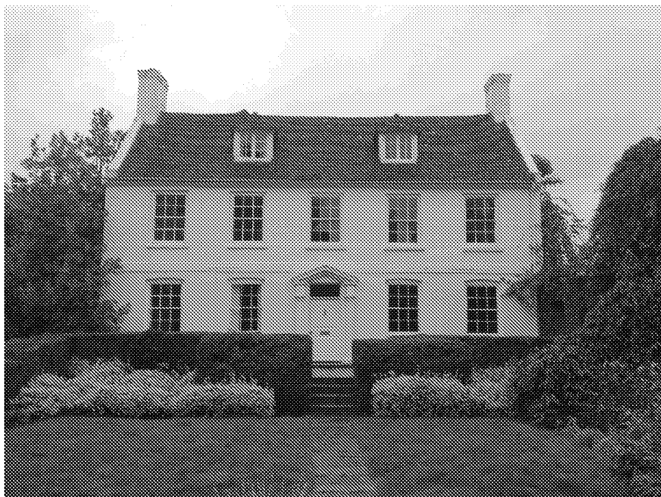
Fig No.1 – Image of Existing Front Elevation
